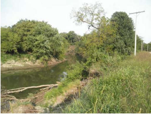
Streambank erosion threatening road and power lines
