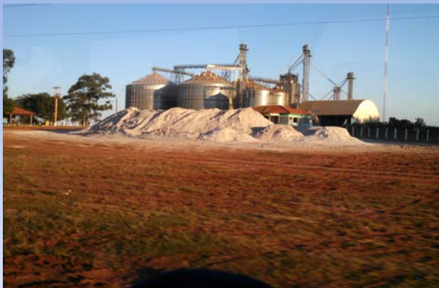
Grain Storage Lime piled on the ground
